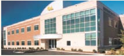
48 Molter Street, Cranston, RI 24,000' Building Ahlborg Family, LLC to Molter St, LLC
