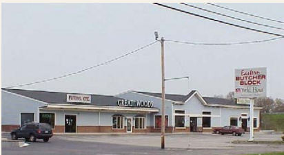
3-5 Progress Street, Seekonk, MA 7,300 square foot retail center Sold to MIS Enterprises, LLC
